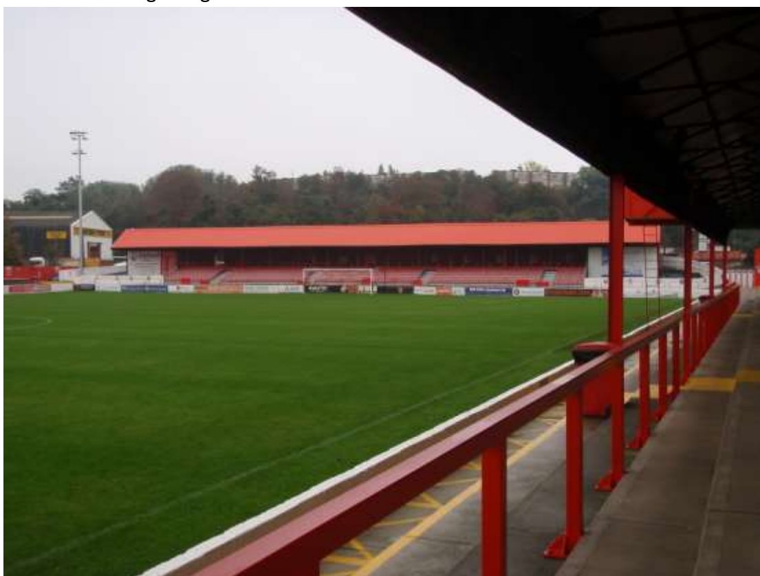
Plate 11. Looking south to the south stand
